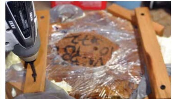
Fixing battens across the burr into the wall to secure the burr in place while the foam sets to the right shape
